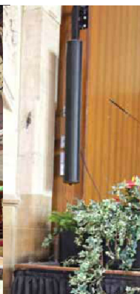
Community ENTASYS 200 column array systems (mounted next to the stone archways) were chosen for the project
